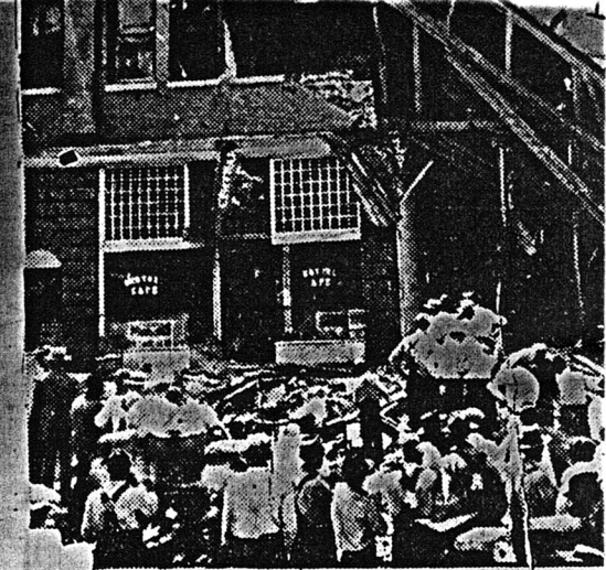
Photo shows general view of workers carrying out dead and injured after nearly one-half of important Shelby, N. C., business block collapsed. The foundations had been weakened.
